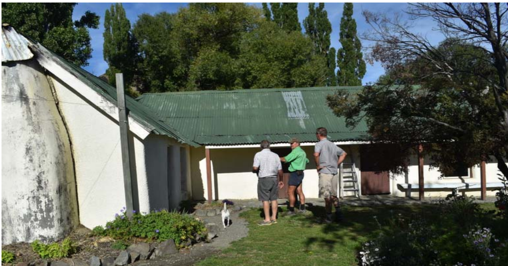
Cob homestead damaged in quake
